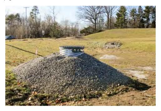
Figure 7-14 Typical Riser Pipe with Stone Jacket
