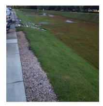
Figure 8-21 Gravel fringe flow spreader
