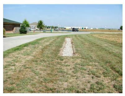
Figure 9-1 Infiltration trench installed adjacent to drive lane
