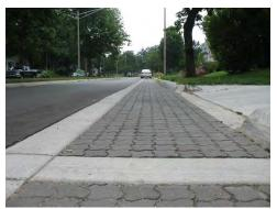
Figure 10-32 Concrete edge restraint between PICP and traditional asphalt
