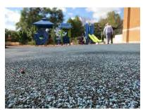
Figure 10-9 Example Rubber Overlay
