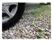
Figure 10-7 Example of Open Graded Aggregate as a Pavement Surface
