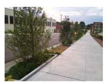
Figure 8-17 Vertical curbing adjacent to sidewalk
