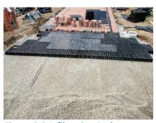
Figure 9-3 Infiltration Bed
