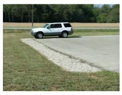
Figure 9-5 Infiltration Trench
