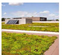
Figure 12-22 Concrete paver paths for maintenance access
