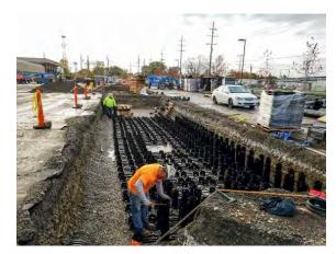
Figure 15-2 Installation of soil cells
