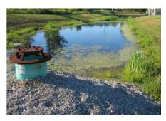
Figure 1-3 Retention basin with outlet riser
