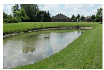
Figure 7-6 Detention with a Permanent Pool
