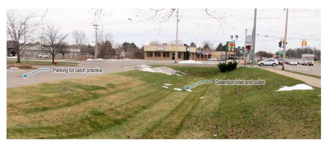
Figure 7-4 Example detention practice with inlet and outlet as the same structure
