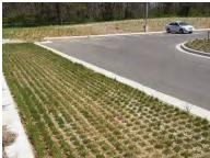
Figure 10-6 Example of Grid Pavement Systems
