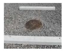
Figure 8-26 Permeable aggregate parking lot outlet structure
