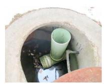
Figure 10-26 Upturned underdrain with a capped tee connection
