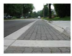
Figure 1-5 Permeable concrete pavers
