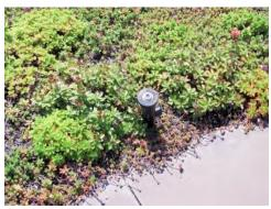
Figure 12-21 Overhead spray irrigation on vegetated roof
