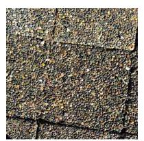
Figure 10-8 Example of Pervious Paver
