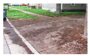
Figure 10-16 Permeable pavement with significant leaf litter
