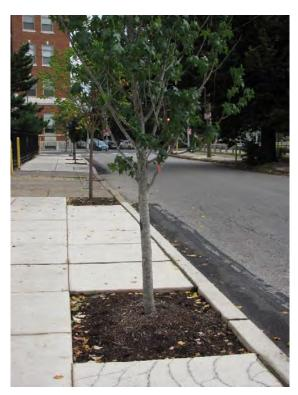
Figure 8-6 Suspended Pavement Sidewalk
