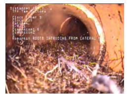
Figure 15-15 Example root growth in sewer
