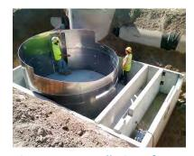
Figure 9-13 Installation of typical manufactured treatment device
