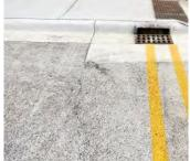
Pervious concrete parking; overflow conveyance to combination catch basin.
