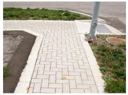
Figure 10-13 Permeable Sidewalk
