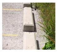
Pervious concrete parking, overflow conveyance to bioretention
