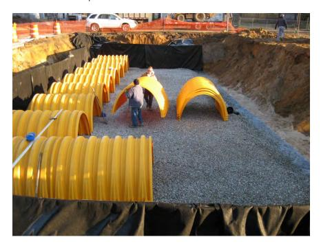
Figure 7-11 Subsurface Detention During Construction
