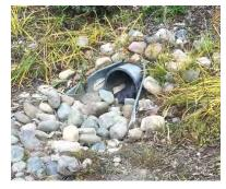
Figure 8-22 Piped inlet
