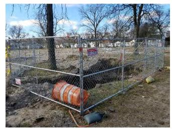
Figure 15-17 Tree protection removed for excavation
