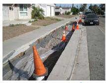
Figure 10-34 Protection of subgrade during construction
