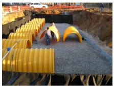
Figure 9-4 Infiltration Vault
