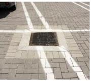
Permeable paver parking; overflow conveyance to flat catch basin inlet.
