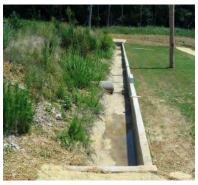
Figure 9-10 Typical level spreader
