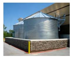
Figure 3-4 Use of cisterns for water reuse
