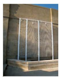
Figure 12-15 Green façade wall-mounted trellis system
