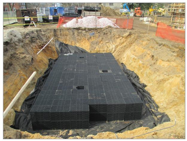
*Installation of an underground plastic grid storage system*
