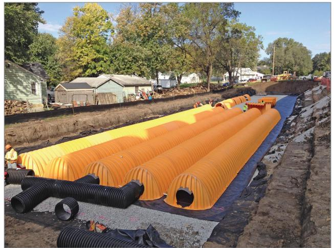
*Installation of an underground pipe and chamber storage system*
